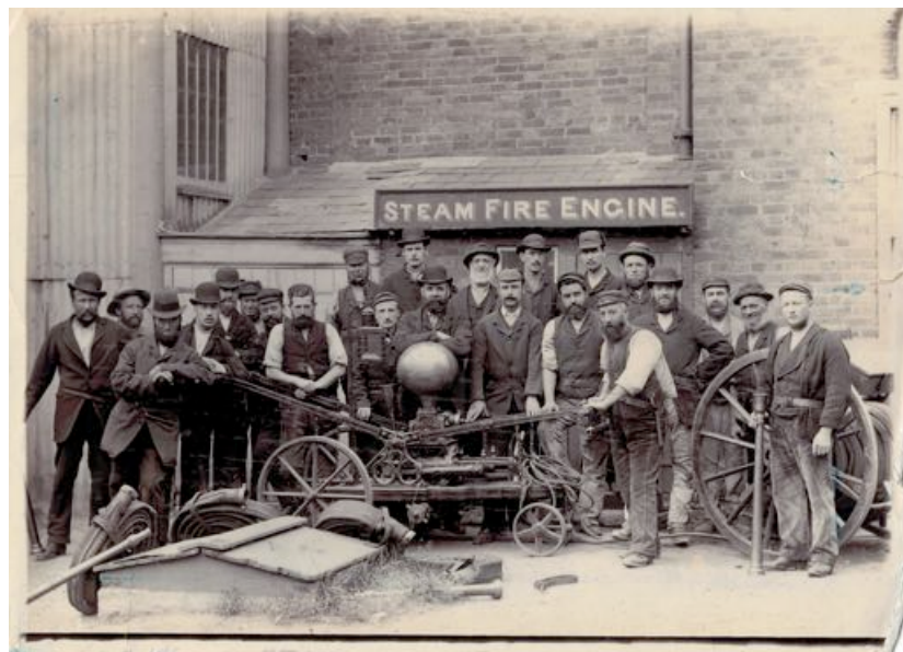
Figure 5: Steam Fire Engine at the Linoleum Works in 1880.
